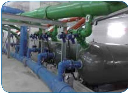
12 Micron MD6500 Commercial fiberglass filters and 11 Micron M5000 Commercial fiberglass filters purify over 4 million gallons of water at Asia's premier destination resort, Universal Studios on Sentosa Island in Singapore. The Micron M5000 filters are used for the water theme park (9,900m<sup>3</sup> volume of water), while the Micron MD6500 filters are installed to service three different attractions,
