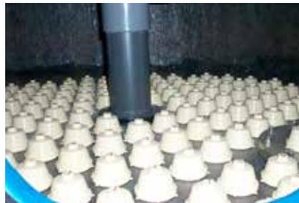
Nozzle Plate under drain system
