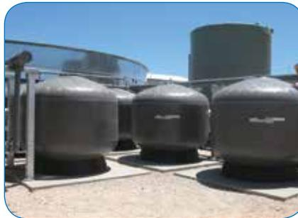
This was a multi-staged project to deliver high quality filtered drinking water to the state's rural and remote communities. Waterco was instrumental in this initiative, installing 8 Micron SMDD2200 Commercial fiberglass filters and 17 Micron SMDD2500 Commercial fiberglass filters filled with granular activated carbon to remove unwanted taste and odours during final filtration stages.
