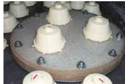
Internal Nozzle Plate Service Hatch
